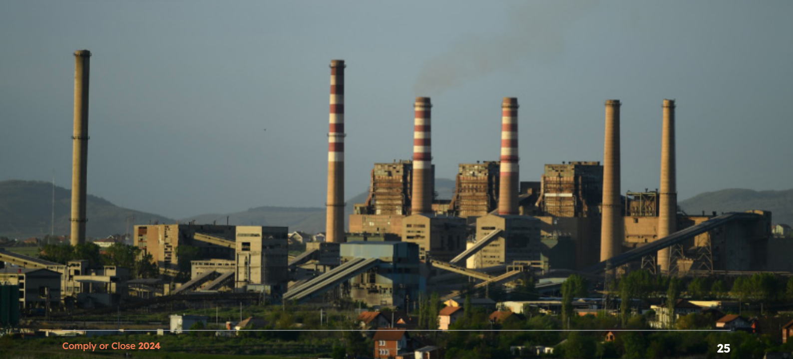
Kosovo A power plant, Kosovo Photo: Arben Llapashtica
